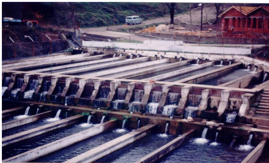
Figure 32. Concrete raceways for fingerling culture
