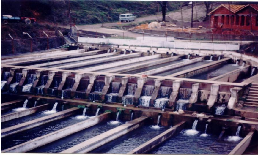
Figure 32. Concrete raceways for fingerling culture
